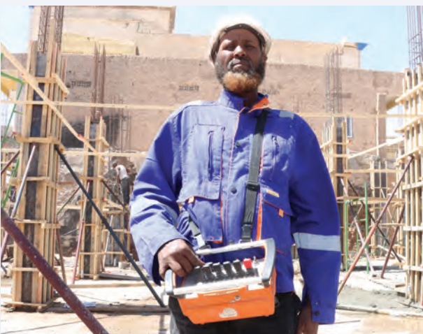
Pharo Construction employee rebuilding the Waheen Market that was hit with massive fire on April 1 st , 2022. The market is located in Hargeisa, Somaliland.
