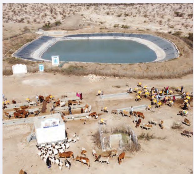
Aerial footage of Illinta dam (75.5mX57mX4m) located in Gabiley, Somaliland. With storage capacity of 17,400.00 cubic meters that will provide clean and adequate water for 247 households through the year particularly during the dry season.
