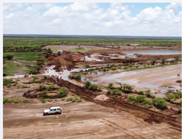
Aerial footage of the construction at the Wado-Makahiil dam, located in Maroodi-Jeex, Somaliland
